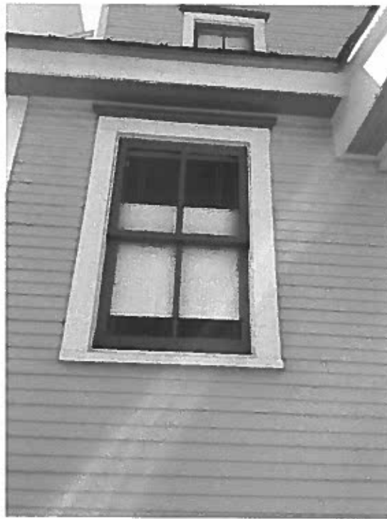
Photo 37: Kitchen Window facing east.
