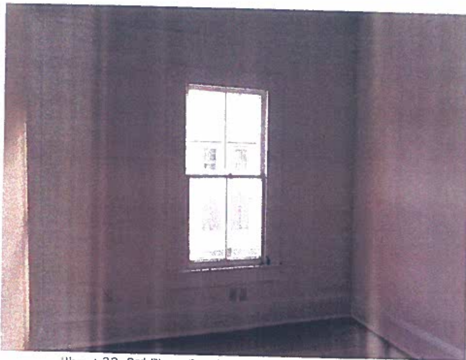
Photo 23: 2 nd Floor South West bedroom facing south
