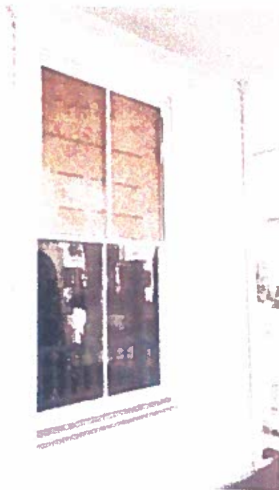
Photo 26: 1 st Floor porch center window. Window faces north.
