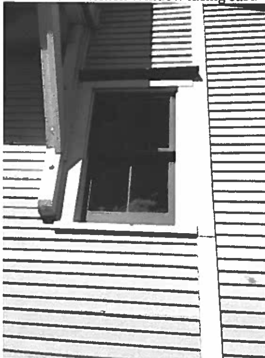
Photo 38: 1 st floor kitchen window facing south.
