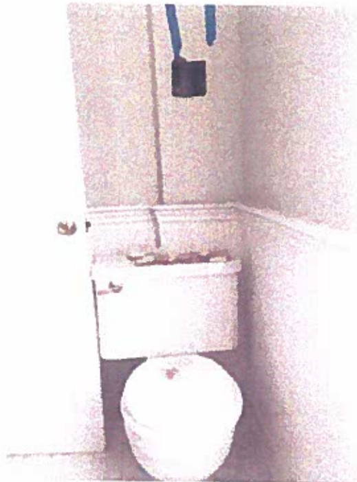
Photo 14: Second Floor East Bathroom facing north
