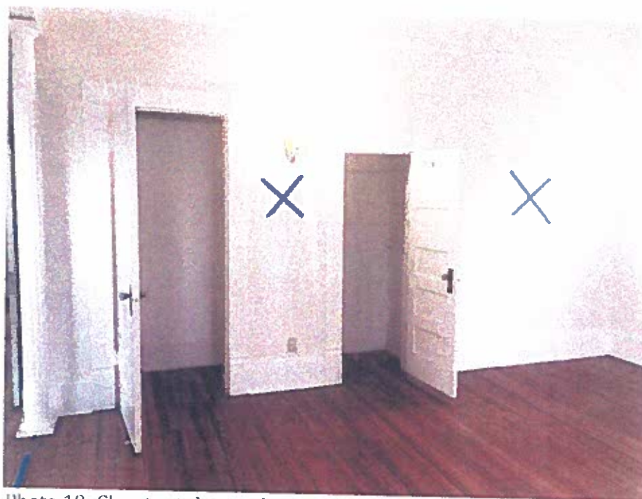
Photo 19: Closets at the southern wall of the 2 nd floor north-west room.
