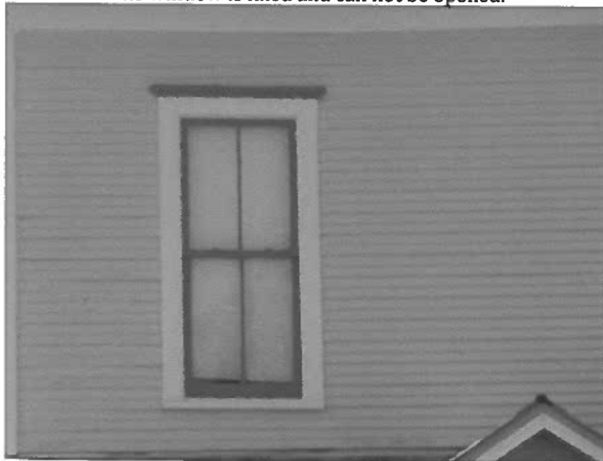
Photo 42: East facing window to the 2 nd floor southeast bedroom.
