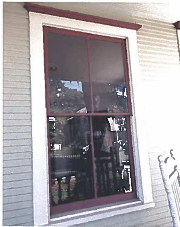
Photo 26: 1 st Floor porch center window. Window faces north.
