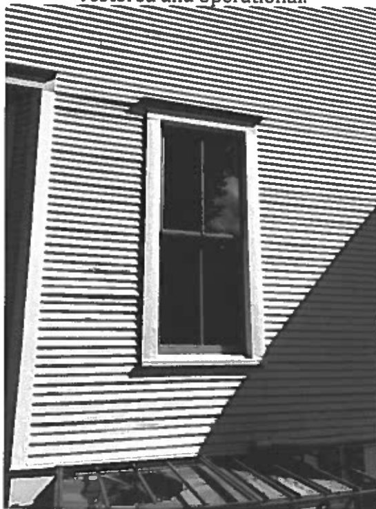
Photo 28: 1 st Floor window facing west. Window restored and operational
