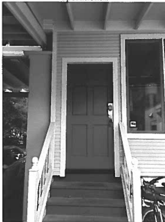
Photo 54: Backdoor at the south side of the house. The door is currently a functional off the shelf door. It is repainted.
