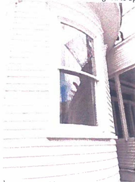
Photo 30: Curved window on west-side turret facing west. Window is painted shut not designed to open.
