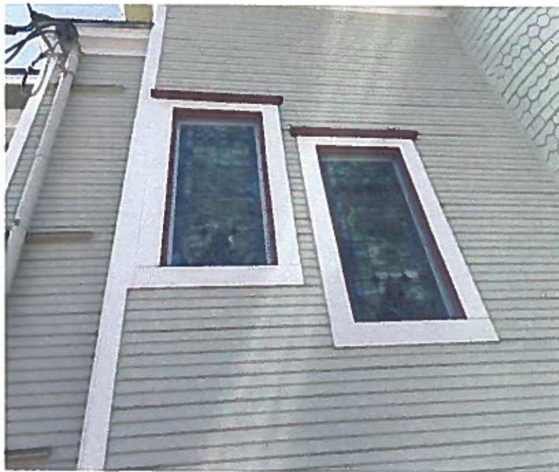
Photo 35: Stained glass windows at the east side of the house. These windows are placed at the landing of the stair case between first and second floor. The windows do not open.
