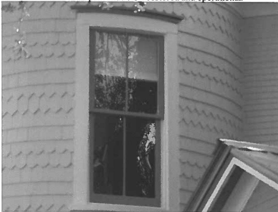
Photo 46: Window on 2 nd floor of turret facing northwest. Window pane was broken and window was paint shut. Restored and operational.
