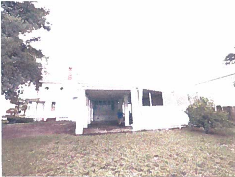
Picture 3: View of east side of 152 East 4 th Street (December 2013)
