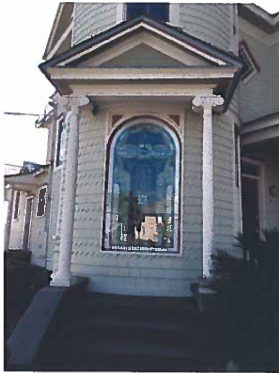
Photo 33: Stained glass window at Northeast corner of first floor. The window is protected by Plexiglas and not designed to be opened.
